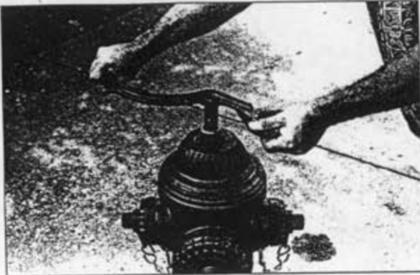
7. Using socket of combination wrench or 3/4" thinwall socket, loosen travel stop nut #5.
