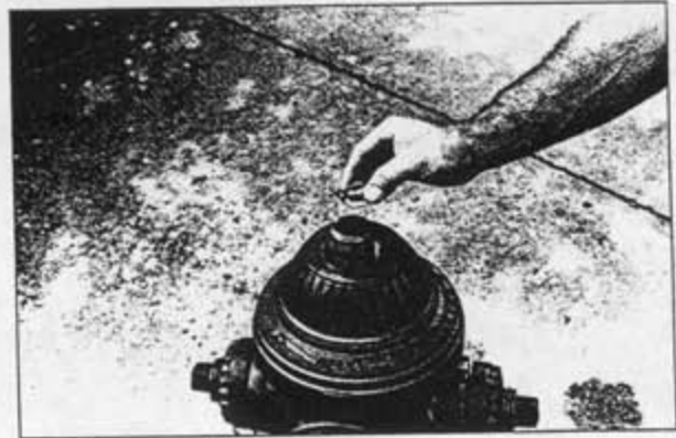
8. Remove travel stop nut #5.
