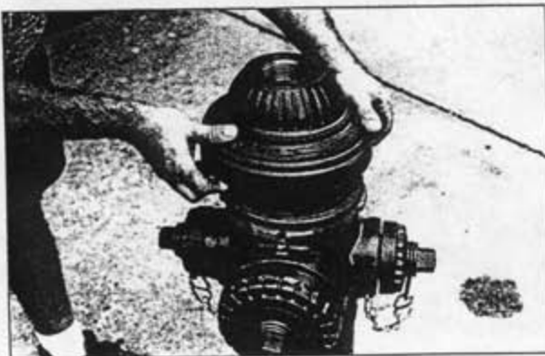
13. Lift bonnet straight up and off the operating rod.
