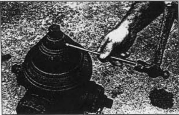
25. Regrease the upper and lower chambers of the revolving nut #13. Replace revolving nut and bearing #47. Replace travel stop nut #5. Replace hold down nut #6 and tighten securely. Tighten hold down nut screw #7. Replace operating nut #1 and pin #3.
