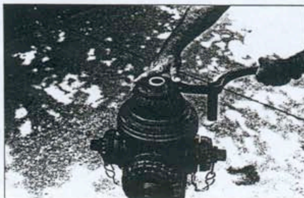
5. Loosen bold down nut #6 using combination spanner wrench by turning counterclockwise.
