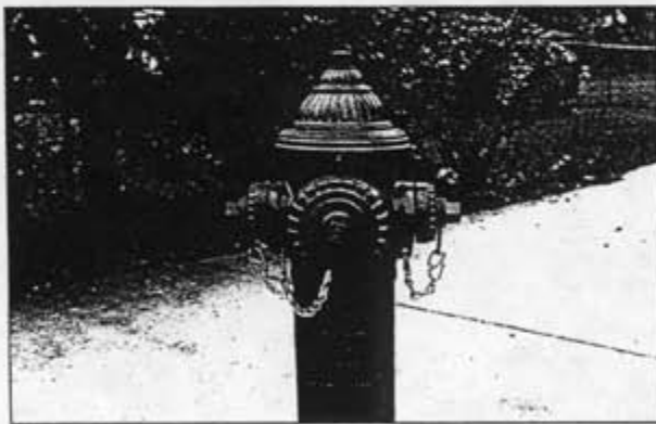
27. Hydrant closed and back in service.
